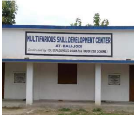
Multifarious Skill Development Center built under CSR at Balijodi, Orissa
