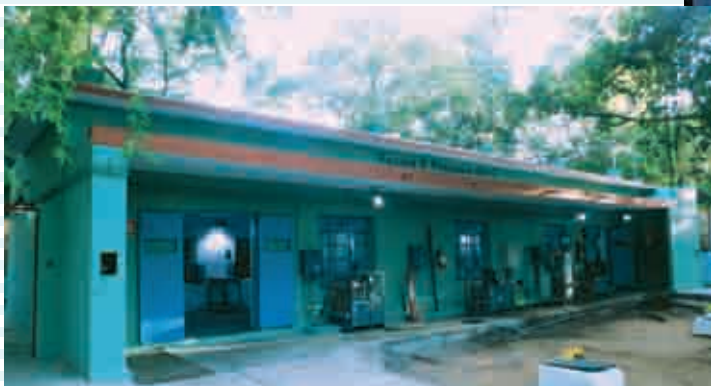
Renovated Filling & Pressing Pant
