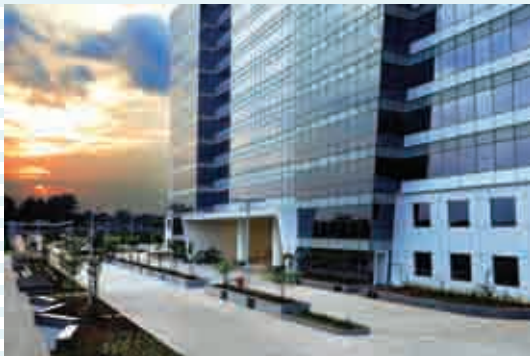
A view of Block 2 Entrance
