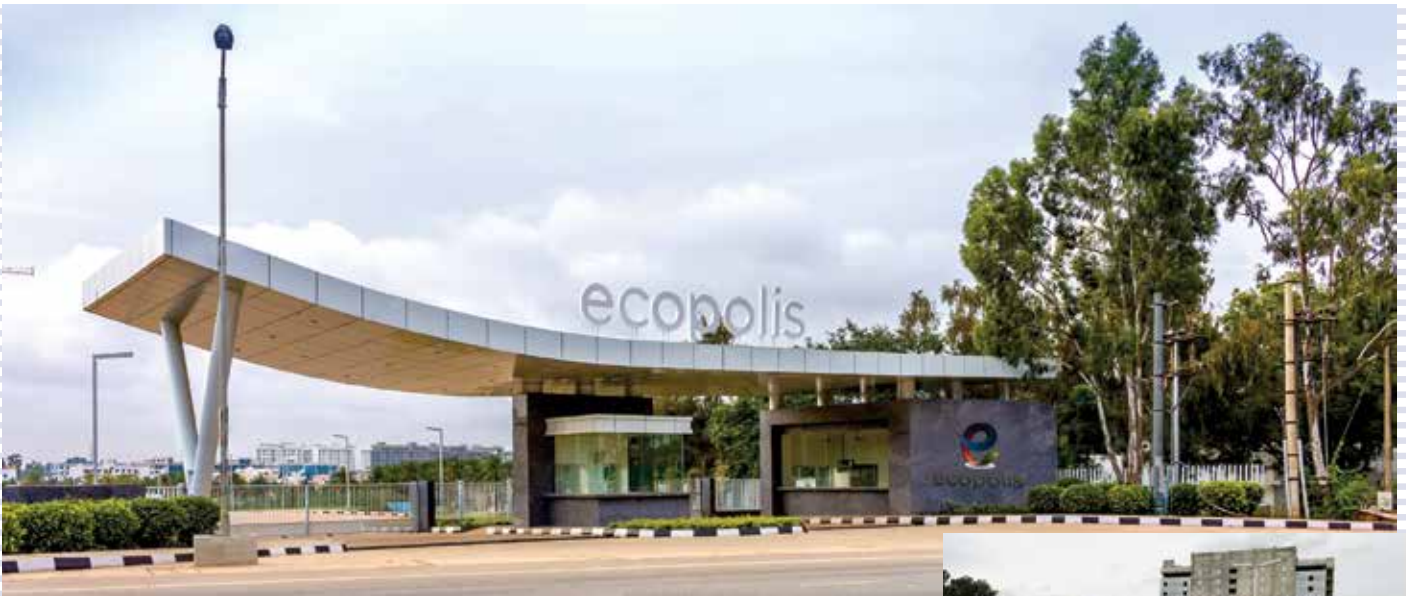
Entrance to Ecopolis
