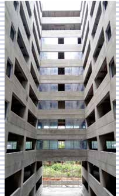
View of passage between 3A & 3B from the lobby
