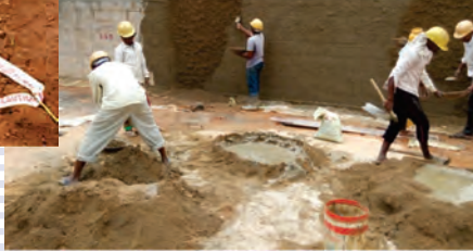
Work in progress at Bengaluru project site
