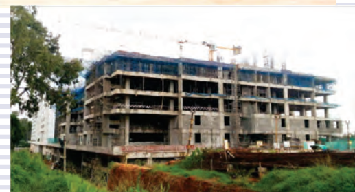
Block 2 under construction
