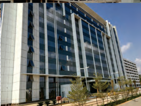
Completed Block 3A & 3B (External)
