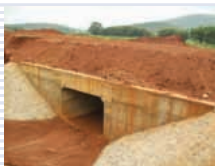
Box culvert on Utkal Alumina India Ltd Tikri Project, Orissa
