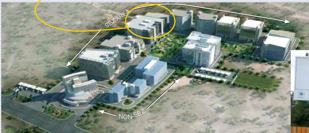
Property Development at Bangalore, First building under construction
